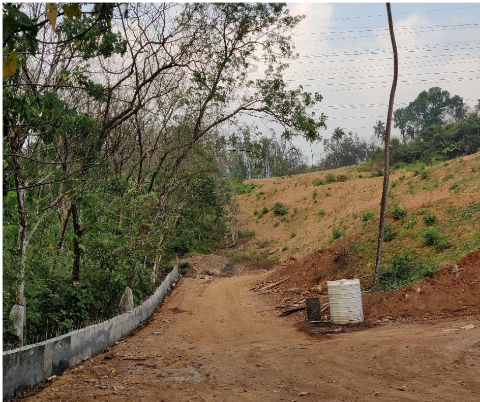
Dumping Area with Retaining wall
